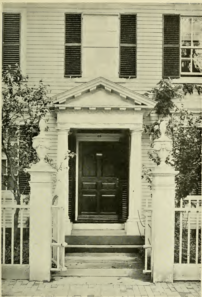
PLATE XC.—Detail of Gateway and Porch, Pierce-Johonnot-Nichols House.
